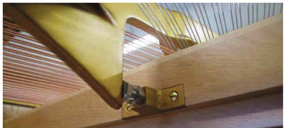
In grand pianos, string tension acts like a “force transducer” at the belly rail and - in accordance with the “circulation principle” - generates a rim tilt via the braces and soundboard compression via the ribs. For this reason, the spruce ribs are positioned against hardwood which increases their life span. On many grands from other piano manufacturers, you can see freestanding, unsecured ribs at the belly rail. The belly rail couples the bass and treble sides.
